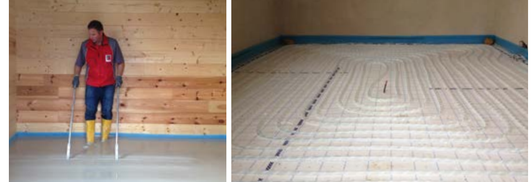
Water-based underfloor heating system in all houses
