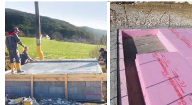
Concrete floor slabs with XPS insulation
