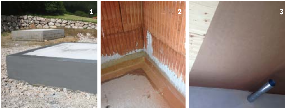
VOC-free base seal (1), VOC-free sealing angle (2), VOC-free waterproofing membrane as a vapor barrier (3)
