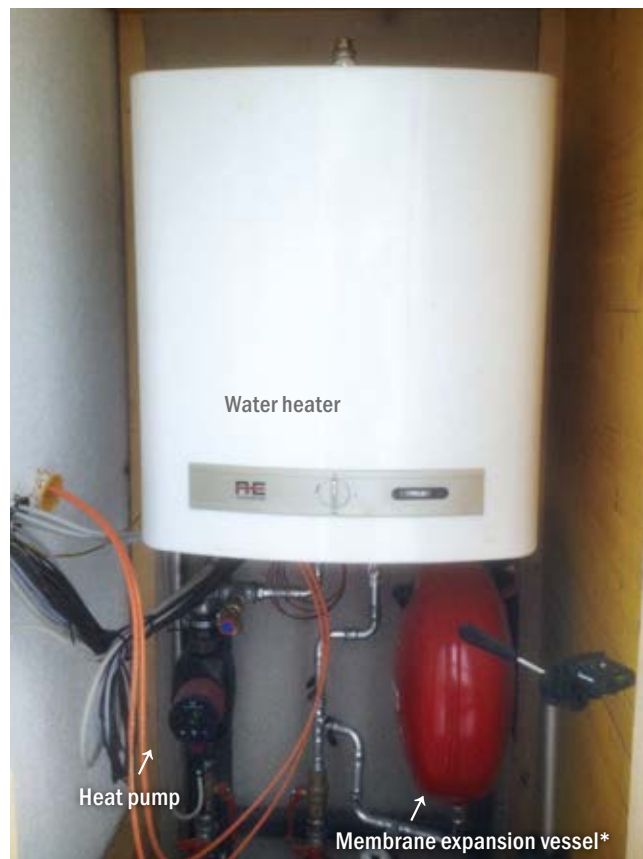
Equipment room with electric water heating
